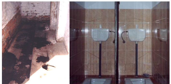
From this wooden hut... to these new ceramic toilets, with many more to come, and at last there are septic tanks – previously the kids themselves emptied the pits with shovels.
